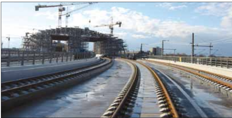
Hauptbahnhof, Berlin Central Railway Station, Berlin
